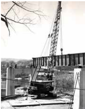
A jib guides a girder into place during construction of Memorial Bridge.
