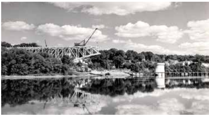
Memorial Bridge begins to take shape in the late 1940s in Augusta.
