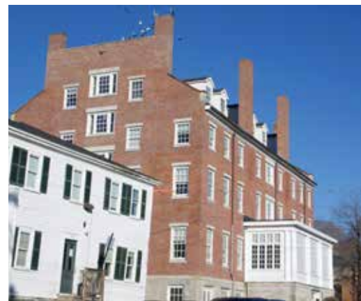
Architect John D. Lord designed Hallowell House and supervised its construction throughout most of 1823 and 1824. It was known in the 20th century as the Worster House.
