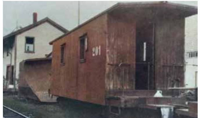
In foreground, a flanger stands beside the railroad tracks decades ago at the Wiscasset, Waterville & Farmington Railway station in Albion.
