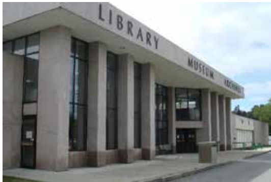
This image shows the Maine Cultural Building in Augusta before renovation began there in 2020.
