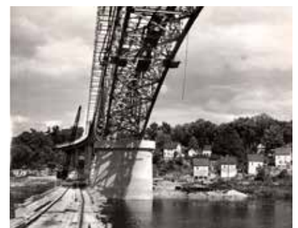
An eastward view shows Augusta’s Memorial Bridge under construction in the late 1940s.
