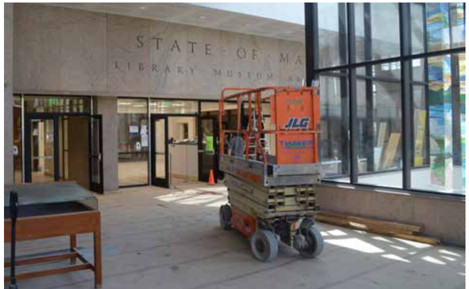
Laborers work to prepare the Cultural Building’s inner entryway May 12 in Augusta in anticipation of the building reopening later this year.
